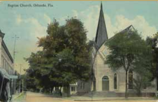
The City of Orlando Building Permits Collection contains a treasure trove of historical details. For example, on July 16, 1913, First Baptist Church trustees applied for a permit to build a frame addition, at a cost of $500, to house the church organ.
