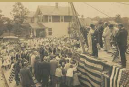
The Board of Public Instruction pulled a permit on June 9, 1917, for a two-story, brick school building to cost $31,417. Contractor F.A. Peppercorn was hired to construct the building in Ramsey’s Subdivision on Central Avenue. Ironically, the building burned in 1973, destroying the existing copies of the building permits that had been stored there.
